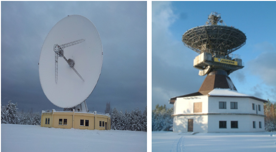
Fig.1. VIRAC radio telescopes RT-32 with antenna diameter 32- m (left) and RT-16 with antenna diameter 16 m.
